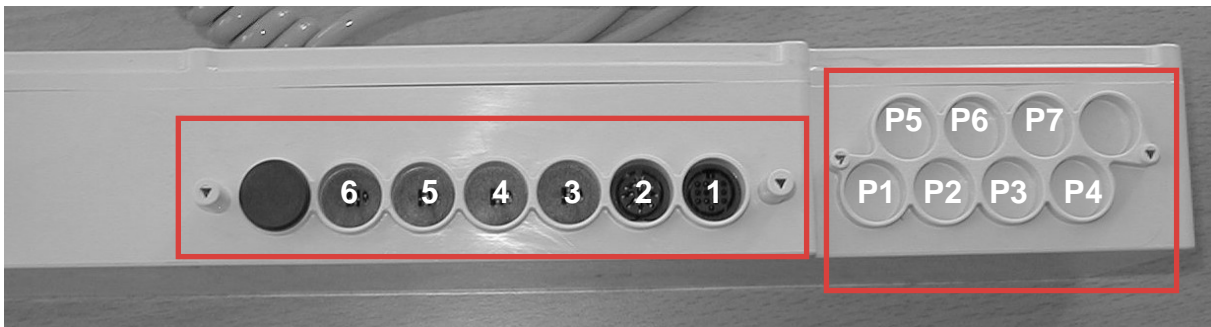
Picture nr. 8: Connection of motors and controls to power box PB 29
